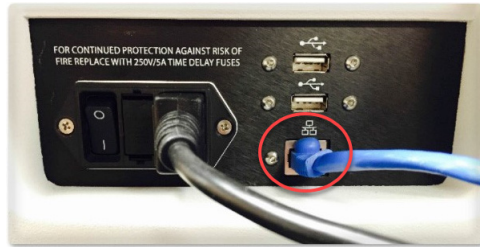
Figure 30. Ethernet port with wired network connection cable
