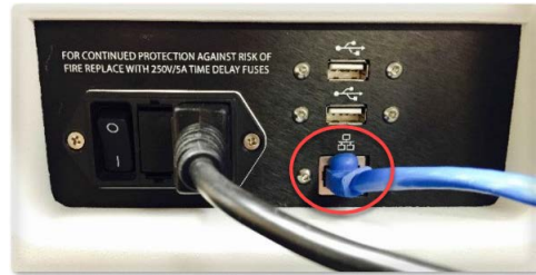
Figure 31. Ethernet port with wired network connection cable
